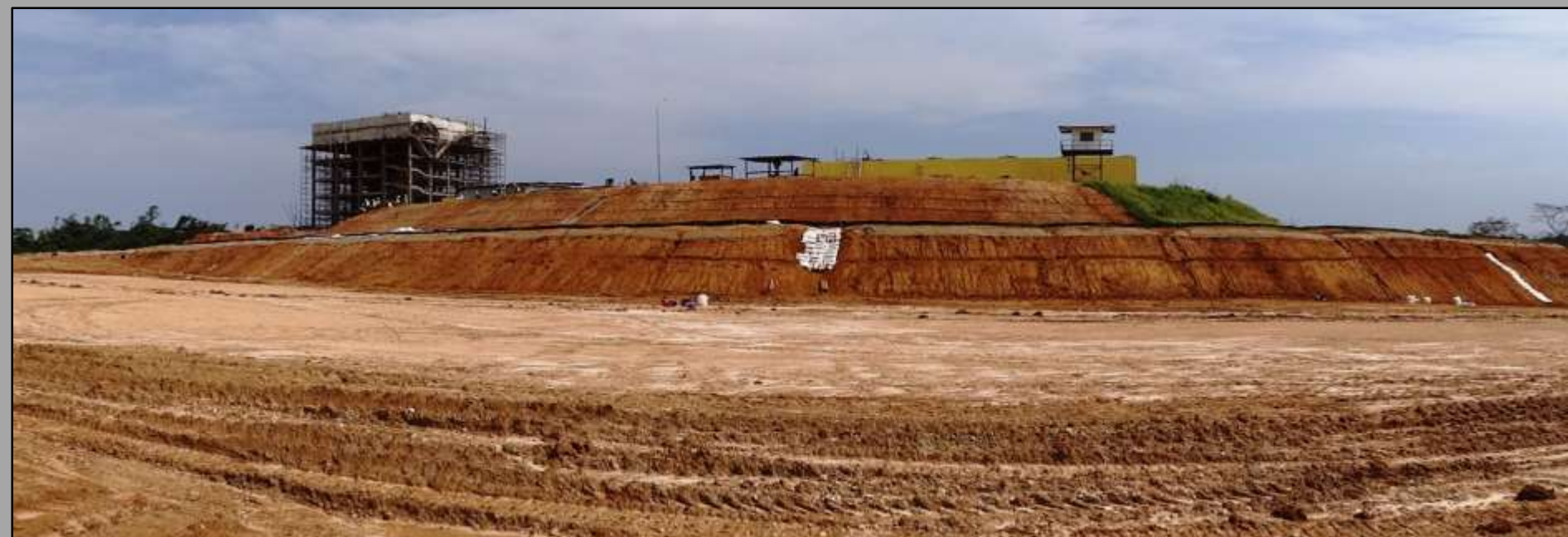
Progressive stages of slope stabilisation using Vetiver (VS), Sand bags, Silt fences & Hydroseeding
