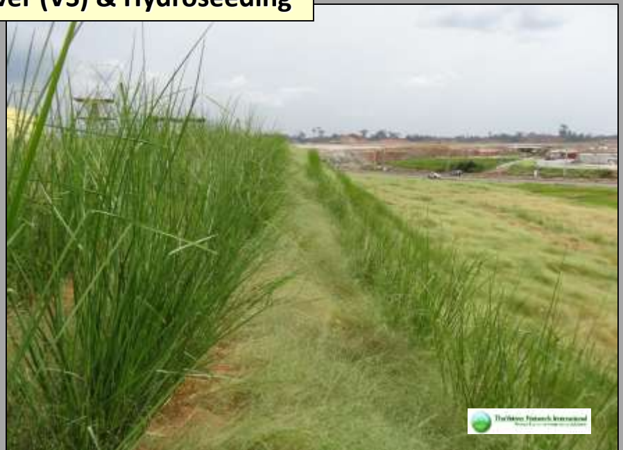
Established Side Slopes using Vetiver (VS) & Hydroseeding
