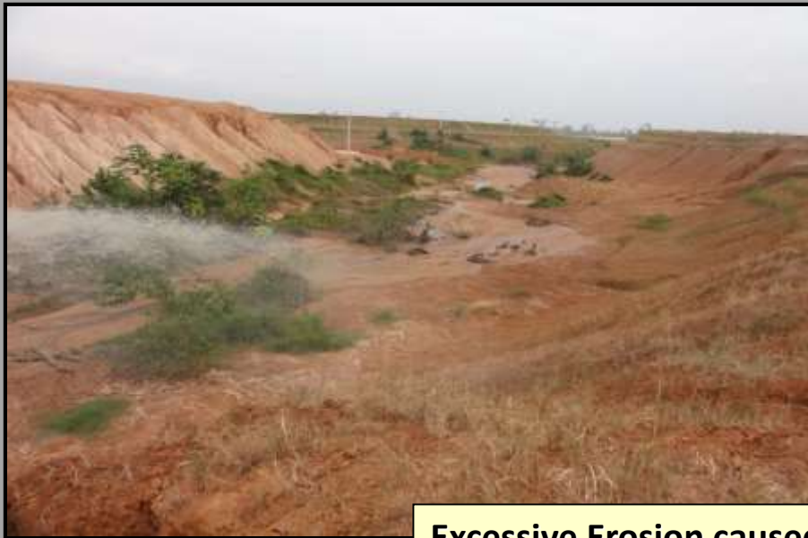
Excessive Erosion caused by surface water runoff
