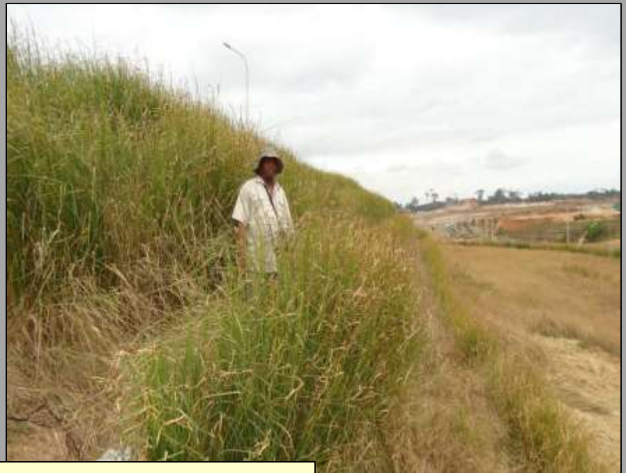
Established Side Slopes using Vetiver (VS) & Hydroseeding
