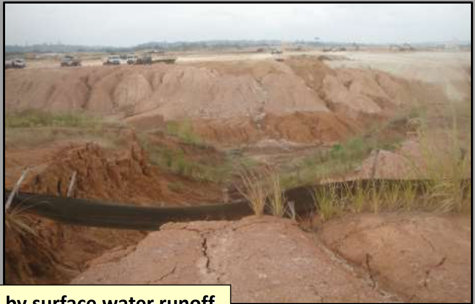
Excessive Erosion caused by surface water runoff
