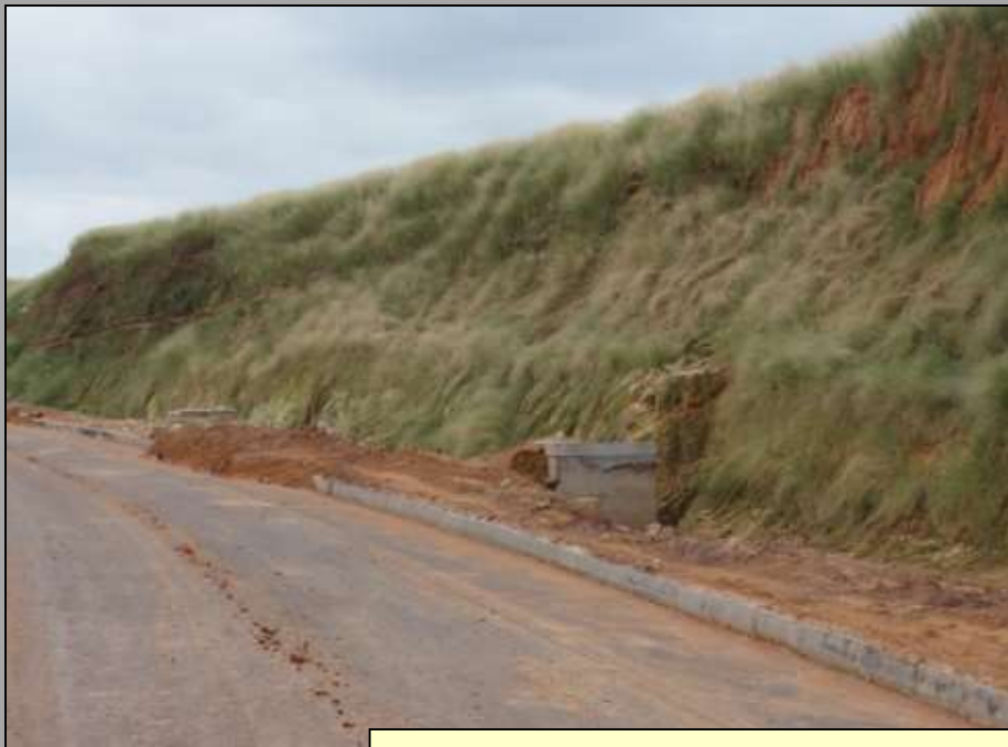
Established Side Slopes using Vetiver (VS) & Hydroseeding
