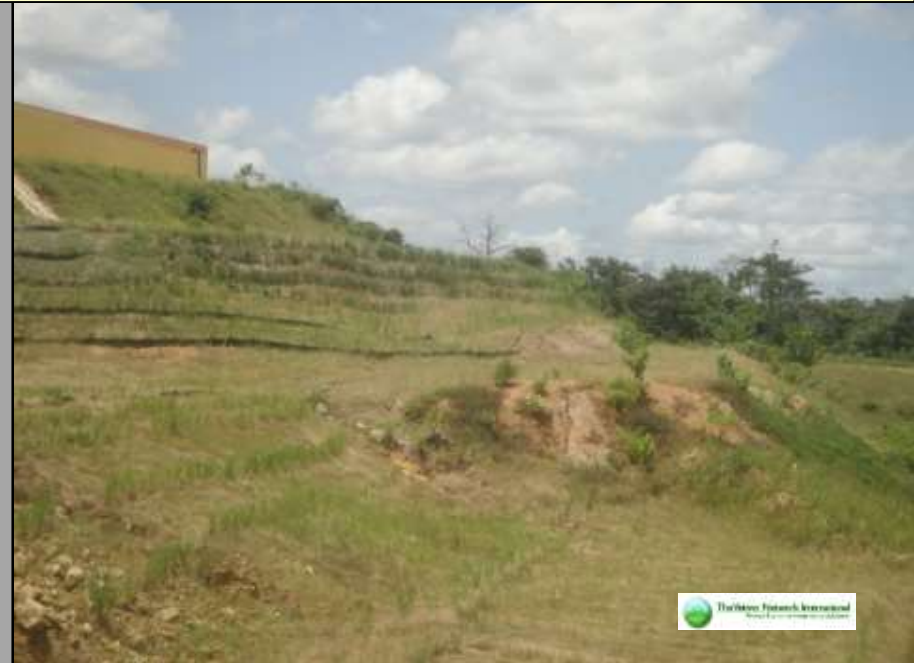
Progressive stages of slope stabilisation using Vetiver (VS), Sand bags, Silt fences & Hydroseeding
