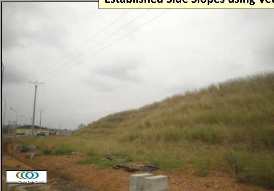
Established Side Slopes using Vetiver (VS) & Hydroseeding
